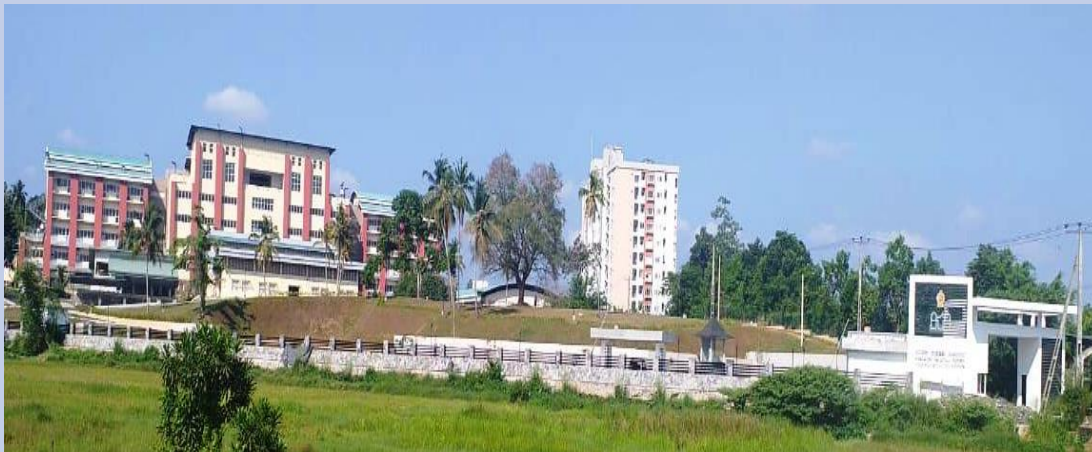
Modern Research and Development Complex, Malabe
